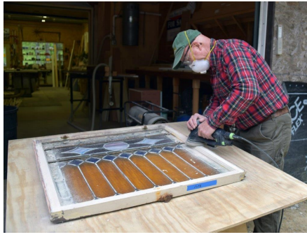
The stained-glass window refurbishment took several steps to complete; to the left, a sash with the old glazing removed; center, a worker sands the layers of paint off the sash; right, the prototype lightbox with the window for the “Rt Rev Bishop”
