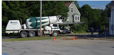
The addition of the ADA ramp makes the museum accessible to everyone. Above left, site work is underway; above center, Coleman Concrete pours the slab for the ramp and sidewalk connecting to the parking lot; above right, a worker is assembling the ramp; left, the finished ramp ready for use
