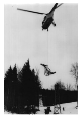
Helicopter hoists chairlift tower
