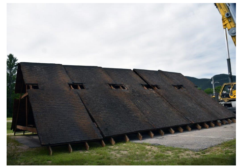
Roof sections rest in the parking lot
