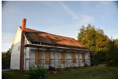
Prepped and ready for the roof removal
