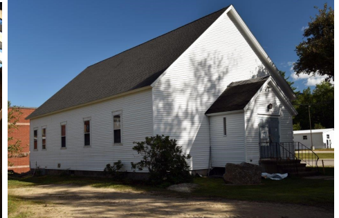
New main roof complete
