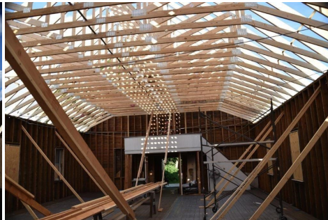
Trusses installed looking to choir loft
