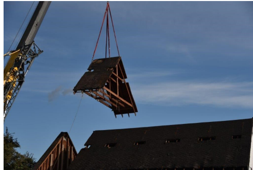
Crane removes the first section of the roof
