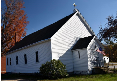
Building before the roof work
