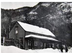
Carrigain Dwelling/Willey House Post Office #2— Photo from late 1800’s
